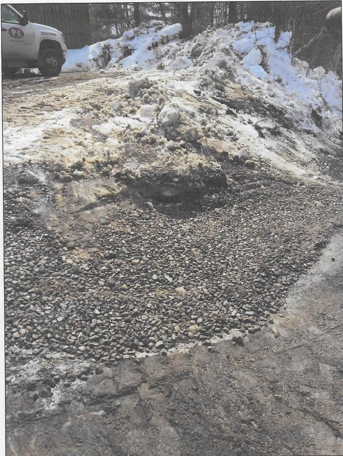
Photograph 6: Gravel backfill.
