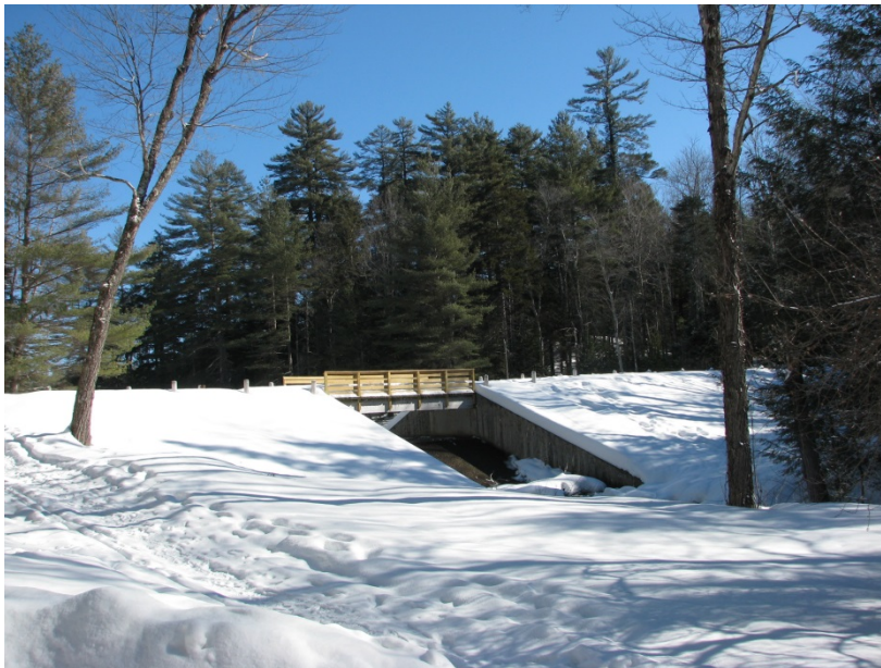
Lowell Lake dam and bridge
