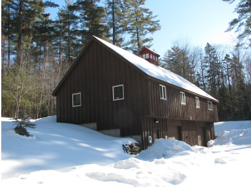
Ranger's residence/maintenance building on Little Pond Road
