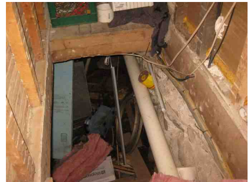
Access to partial basement
