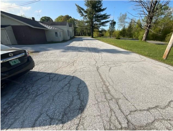
1 - OVERVIEW OF ACCESSIBLE PARKING AREA
