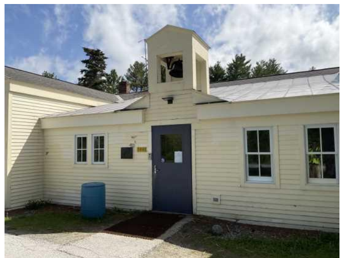
6 - MAIN BUILDING ENTRANCE
