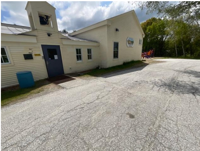
10 - ACCESSIBLE ROUTE TO PLAYGROUND
