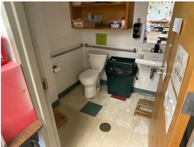
8 - TOILET STALL OVERVIEW
