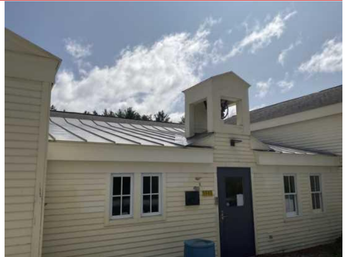
8 - SECONDARY METAL ROOF OVERVIEW
