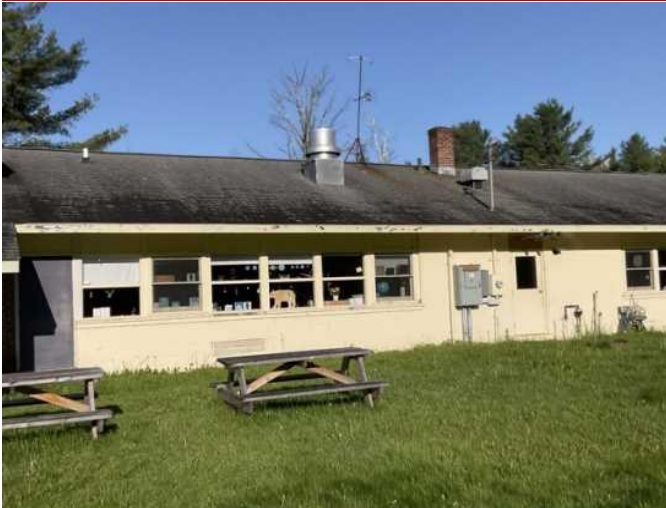
7 - PRIMARY ASPHALT ROOF OVERVIEW
