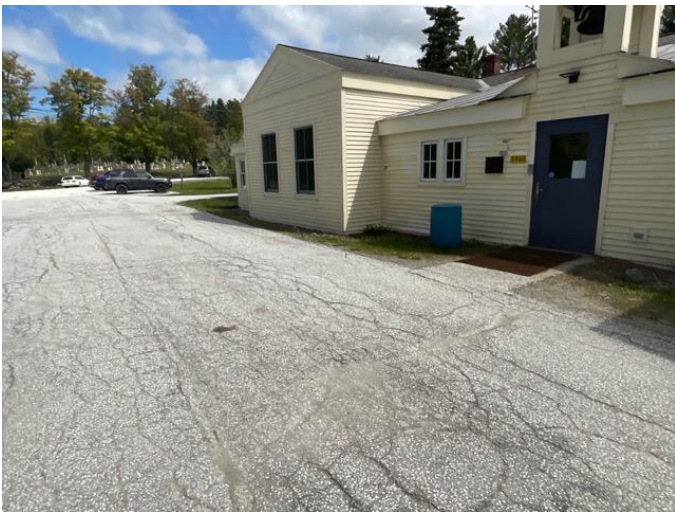
3 - EXT RAMP or PRIMARY PATH OF TRAVEL
