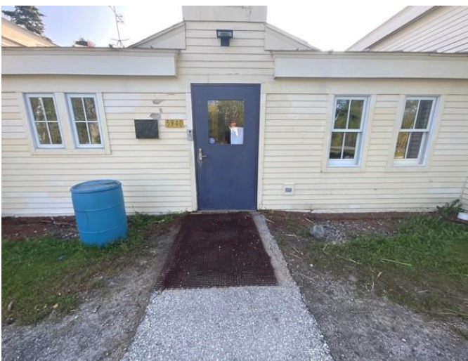
5 - FACADE IN FRONT OF BUILDING
