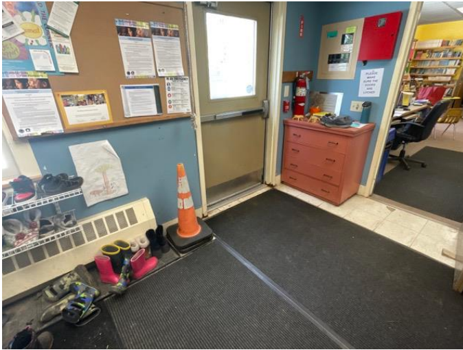
6 - ACCESSIBLE INTERIOR PATH (RAMP/LIFT)
